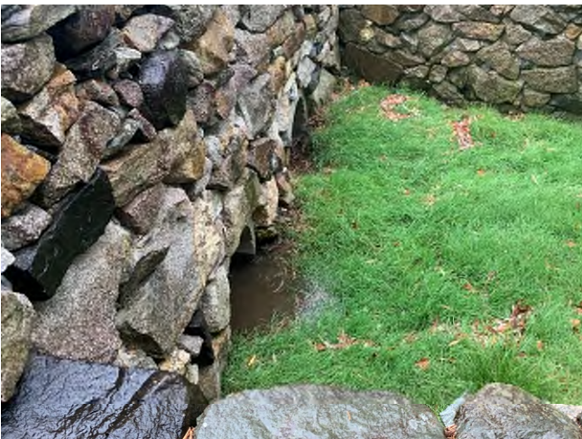
4 Brickyard Circle - 1 (Drainage Course)
