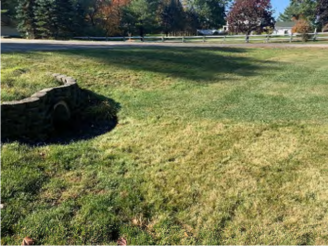
29 Gundalow - 1 (Drainage Area)
