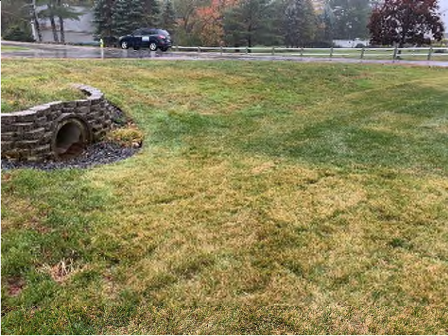
29 Gundalow - 1 (Drainage Area)
