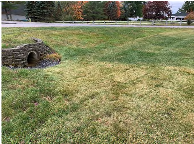
29 Gundalow - 1 (Drainage Area)
