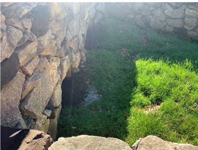
4 Brickyard Circle - 1 (Drainage Course)
